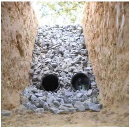
French Drain with two perforated pipes. Rounded gravel is preferred, rather than the angular crushed gravel (as shown)
